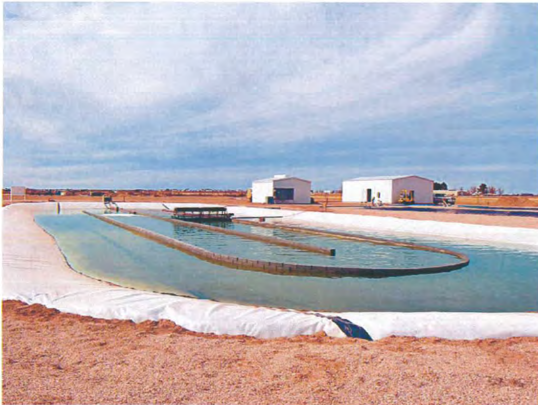
Figure 1. CEHMM outdoor raceway pond and buildings which house extraction equipment
